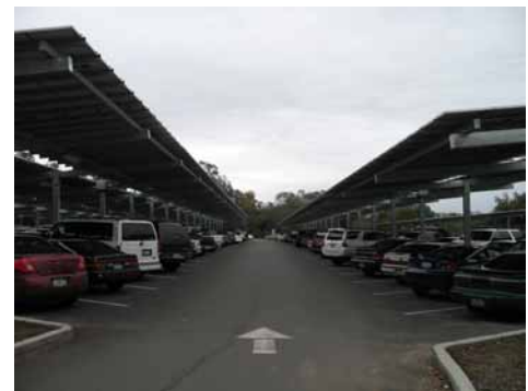
PV Panel Structures
